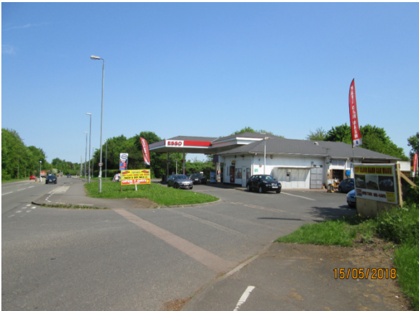
View of the site from the south.
